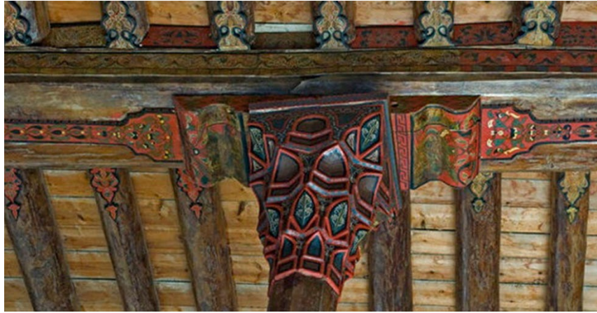
Figure 12 Eşrefoğlu Mosque wooden sleepers and wooden column capitals
