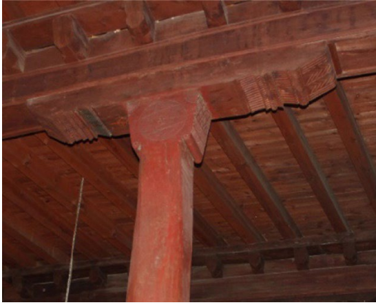
Figure 10 Üzümlören Great Mosque wooden sleepers and wooden column capitals
