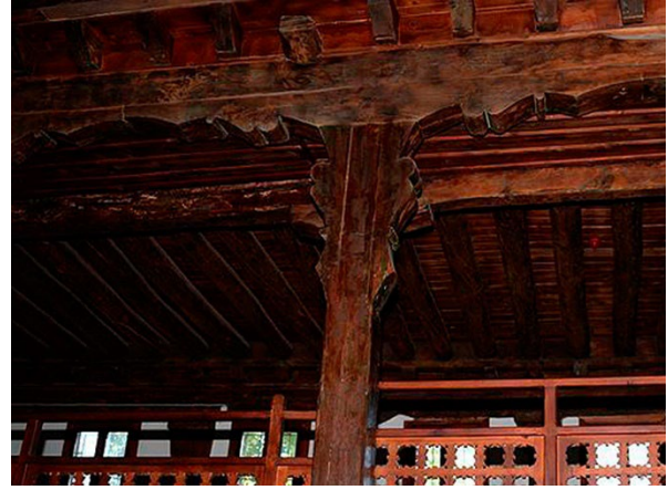
Figure 11 Malum Seyit Mosque wooden sleepers and wooden column capitals
